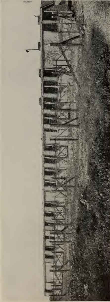
A modern California poultry house. Observe the large amount of curtain front for the admission of direct sunlight.
